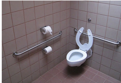
Fully accessible washrooms on all floors.
